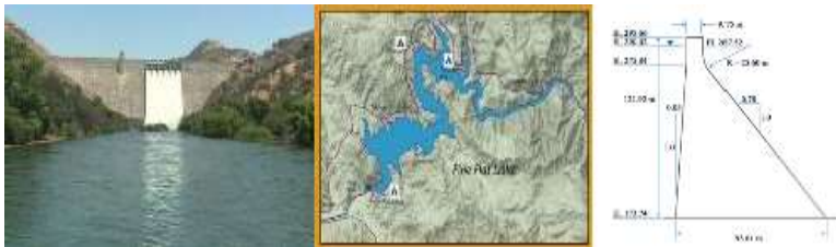
Figure 1. Geometric conditions of Pine Flat Dam (2)
