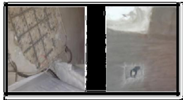
Figure 28: Sacrificial Zinc Anode
