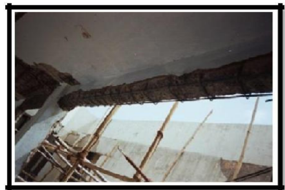
Figure 20: Corrossion of Stirrups
