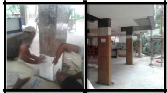
Figure 27: GFRP Wrapping of Columns
