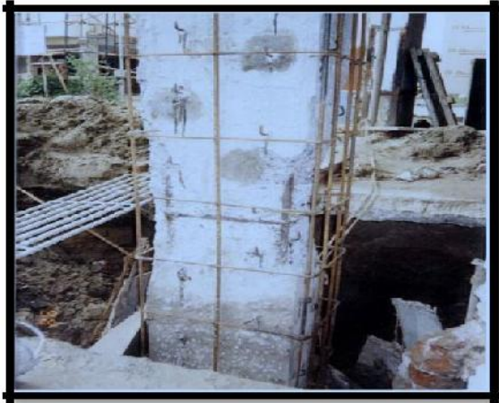
Figure 23: Concrete Jacketing
