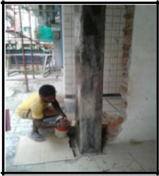
Figure 5: Polymer Surface Coating
