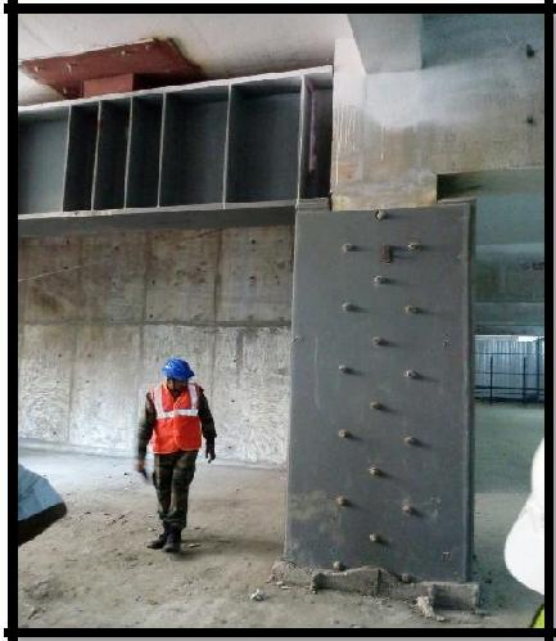
Figure 14: Steel Jacketing of Beam and Column at Trump Tower, Mumbai
