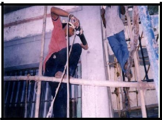
Figure 24: Epoxy Grouting
