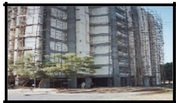
Figure 22: Repair with Polymer Modified Mortar
