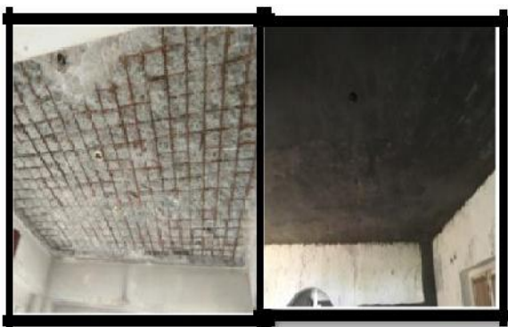
Figure 26: Application of PMM on Roof
